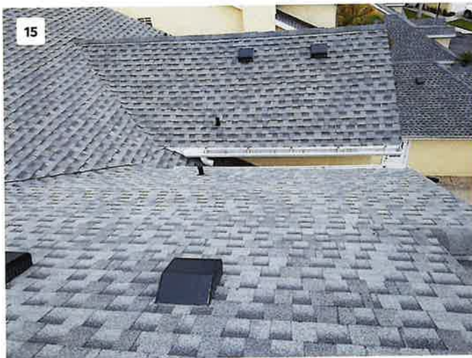
Project: WESTCHESTER SHORES - MASTER / 2407-5882872-01 Date: Jul 15, 2025, 2:49 PM Creator: Lucio Roofer
